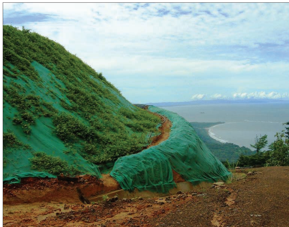
Erosion control techniques, including stabilized slopes and properly lined drainage channels, reduce the amount of sediment runoff, a problem which can be particularly detrimental to rivers and ocean ecosystems.
